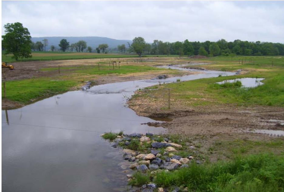
Downstream view of recently completed Oil Creek restoration project showing riparian forest buffer planting and streambank fencing
